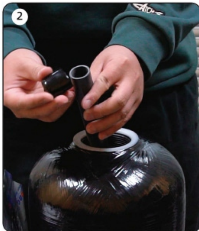
Connect plastic cap to the riser tube and put it in centre of the tank
