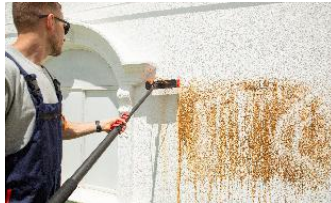
⑧ Commencement of work
