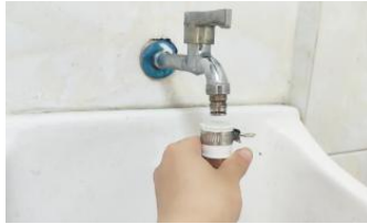
⑤ Connect the white universal water connector to the faucet.
